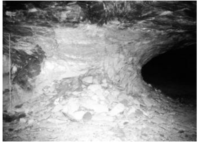
Figure 8: Typical pillar contour damage.
